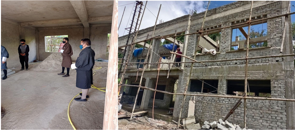
Progress of 32 bedded hostel construction at Buli CS
