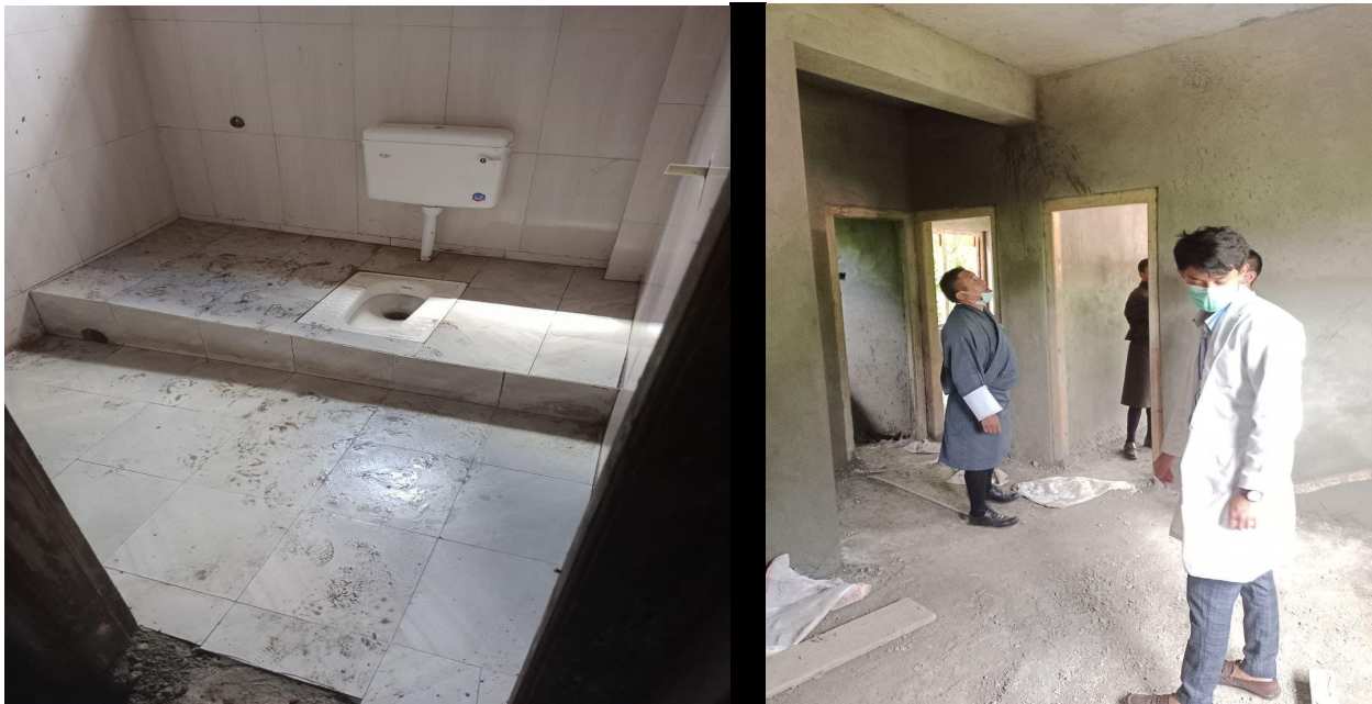
Tiles work finishing at Buli BHU staff quarter construction
