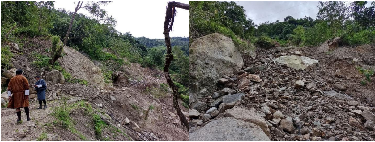
Flooded and landslide area at Zamdong
