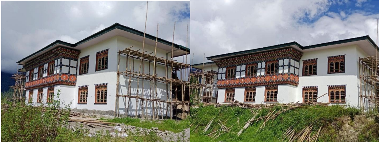
Progress for the construction of 6 unit classroom at Buli CS
