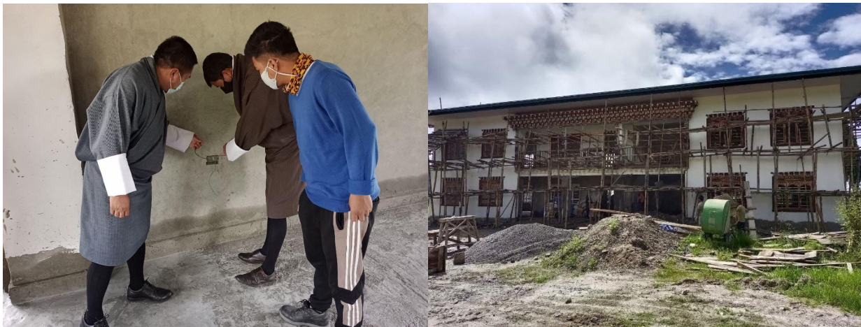
Quality check for electrical wires
