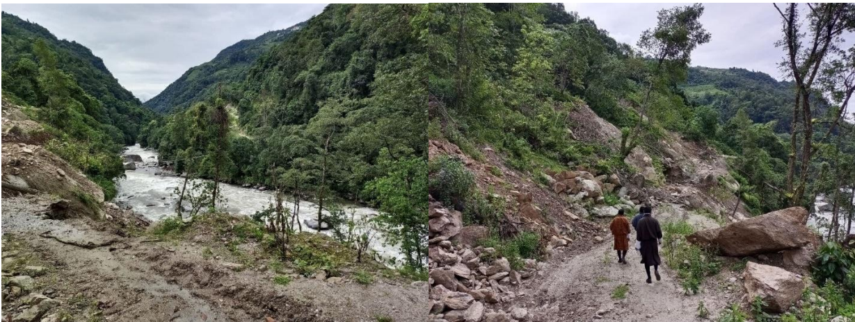
The actual location of the Zamdong bailey bridge construction site
