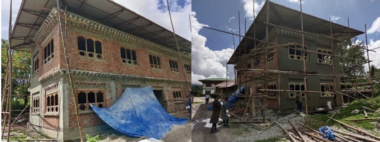
Progress of Buli BHU staff quarter construction
