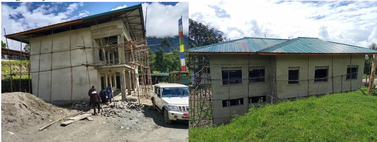
Progress of 32 bedded hostel construction at Buli CS
